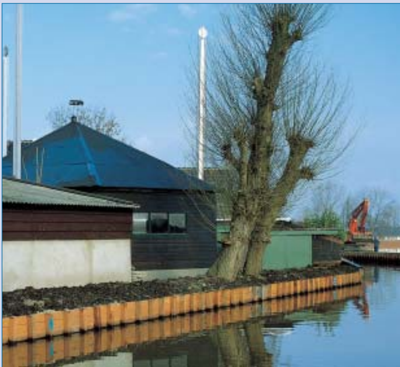
◁ 8. Damwand in bangkirai.
