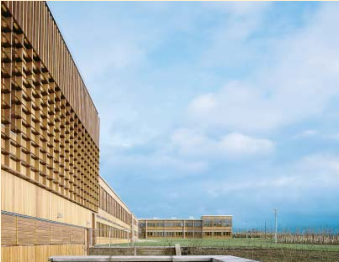
EU Food and Veterinary Office te Grange, Dunsany, Ierland; ontwerp: Office of Public Works Dublin/Ciaran O'Connor. Amerikaans wit eiken in de horizontale gevel-delen en de rasters.
